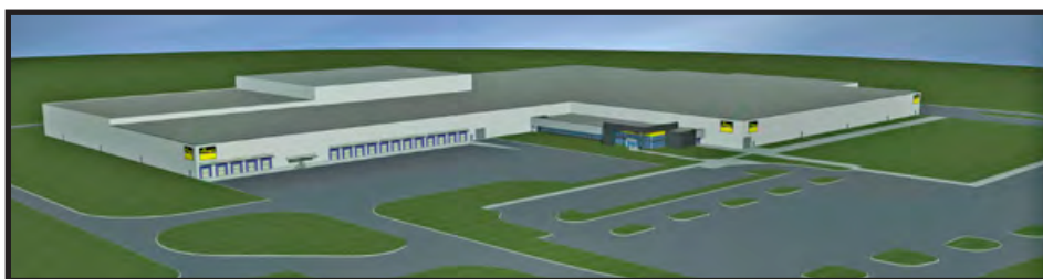
An architect's rendering shows the massive exterior of the new Viega LLC McPherson, KS, facility. At left are the logistics area and loading/unloading docks. The extrusion and injection molding areas are on the right. The view is from the southwest.
