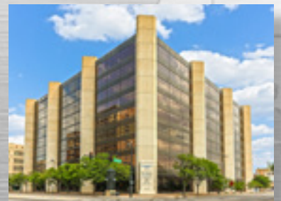
Viega North American Corporate Headquarters Wichita, KS
